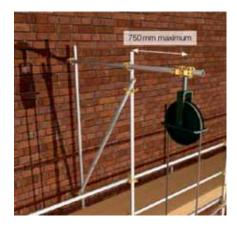
If a joint occurs in an inner standard between the horizontal gin wheel support and the lift below, the joint should be made with a sleeve coupler, rather than a joint pin, to resist uplift. Alternatively, a short section of tube may be spliced across the join and connected with two swivel couplers or band-and-plate couplers.
