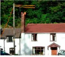
Overhead power lines made safe with shrouding
