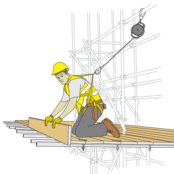
Figure 44: Falling object protection fan erected using an inertia reel.
