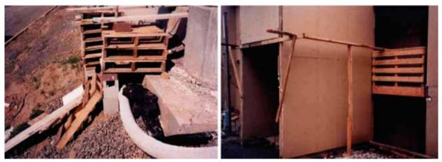
Figure 3 & 4. Loose material, insecure wooden frames, trailing cables etc.
