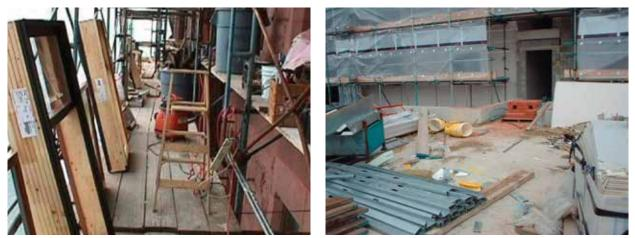
Figure 1 & 2 – Typical pictures of cluttered walkways, uneven scaffold boards, trailing electrical leads etc.
